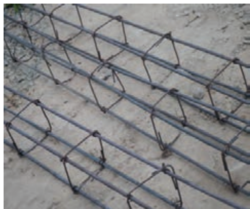
Photo A1: Prepared reinforcement ready for casting ring beam. The size of stirrups used was 6mm instead of 8mm and the spacing was 400mm instead of 200mm in Completion, Construction and Provision of School Facilities at Mboga Secondary School, Bagamoyo DC
