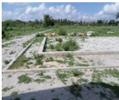
Photo A3: Construction without adherence of drawings for foundation blocks at Majohe Primary School, Ilala MC.
