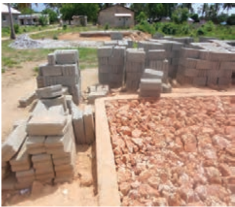
Photo A5: Poor blocks used in construction of Majohe Primary School, Ilala MC
