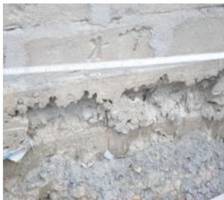
Photo A2: Concrete with Honey Combs at Construction of Labour Ward at Kiwangwa Dispensary, Bagamoyo DC
