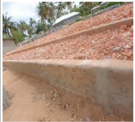
Photo A6: Poor walling including cracks used in construction of Majohe Primary School
