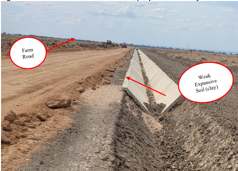
Figure 6: Constructed farm road over weak, expansive soil clay
