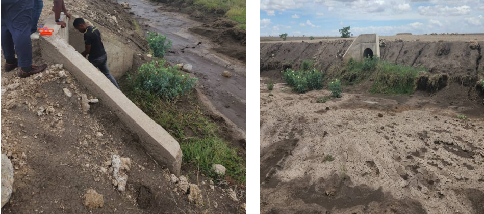
Figure 9: Unsuitable low-quality natural soil
