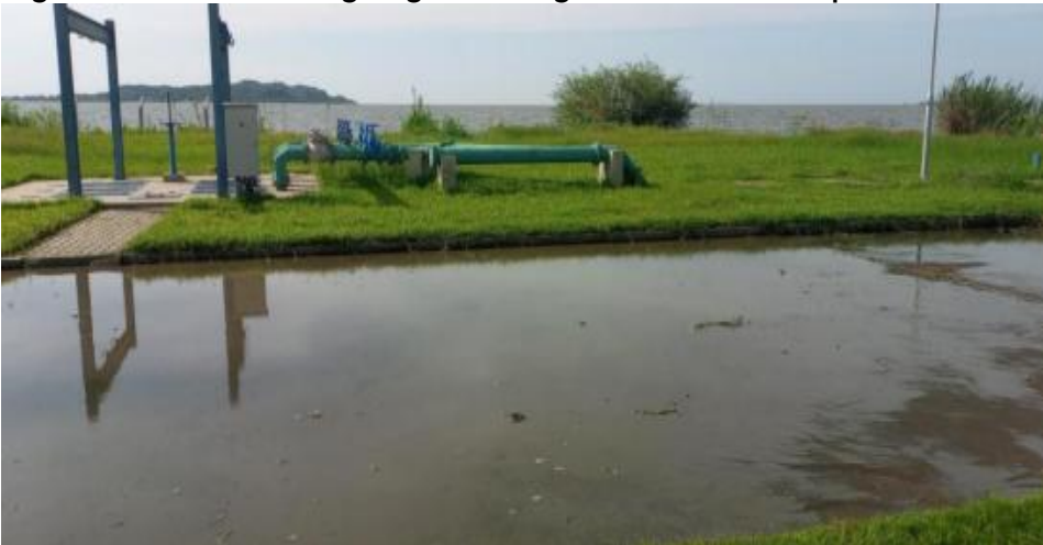
Figure 8: Inundated sludge lagoon at Magu water treatment plant intake
