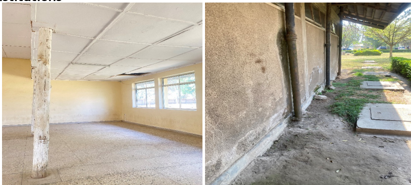
Photo 1: Conditions of Learning Facilities in the Visited Technical Institutions
