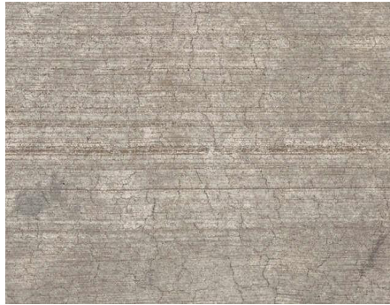
Laitance/Crazing seen at Ch. 4.94 Source: C-Labs Investigation Report.
