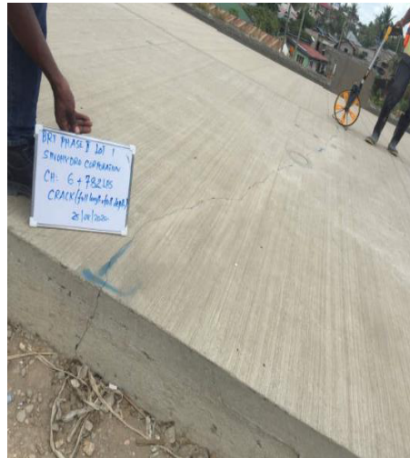
Transverse and Longitudinal cracks (not shown). Photo from Ch.6.780
