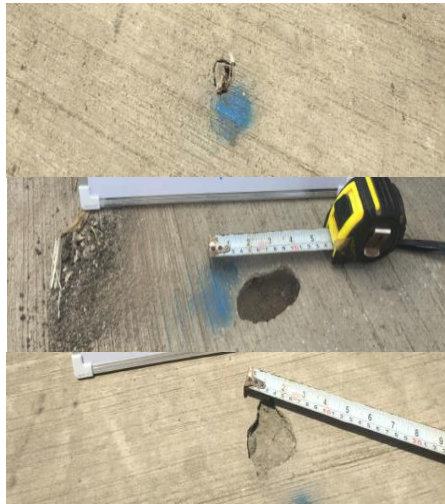
Potholes/Pop outs appearing on all sections
