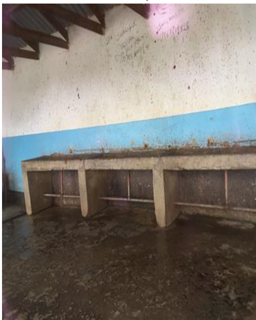
Photo 4 (a): Cattle slaughtering Facility at Makambako with deformed water system for washing internal offal. Photo by auditors on 21 st January 2020 at 01:19 P.M.
