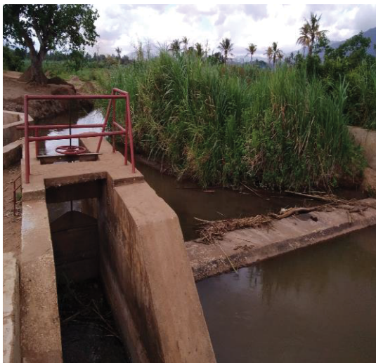
Photo 3.2: Observed siltation at water inlet facilities of the irrigation system due to ongoing upstream activities at Mahenge Ward, Korogwe Town Council (Photos were taken on 02 nd November 2020)
