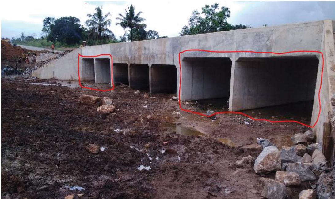
Photo 3.12: Observed part of the Mandra Bridge along Seger-Korogwe Section with added Box Culverts to accommodate the excessive flow of Storm-Water ( Photo was taken on 05 th November 2020 ).
