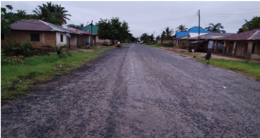
Photo 3.9: Paved tarmac roadway named Matumbi road at Kilwa Masoko in Lindi region. The roadway lacks side-drainages ( Photo was taken on 12 th November 2020 )
