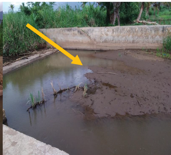
Photo 3.2: Observed siltation at water inlet facilities of the irrigation system due to ongoing upstream activities at Mahenge Ward, Korogwe Town Council (Photos were taken on 02 nd November 2020)
