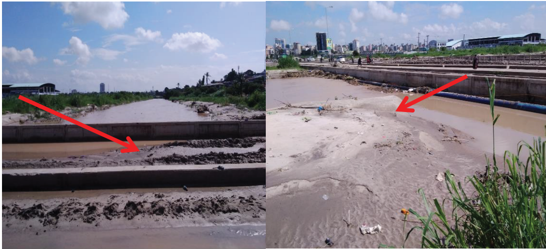
Photo 3.7(c): Observed section of Jangwani Bridge along Morogoro road indicating cumulated sand which comes along Msimbazi river. (Photos were taken on 18 th November 2020)
