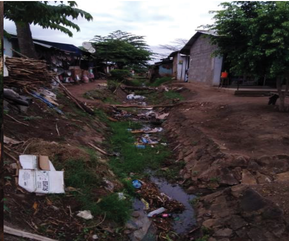
Photo 3.1 (b): Accumulated debris in storm-water drainage nearby the market at Manundu Ward, Korogwe TC (Photo was taken on 03 rd November 2020)
