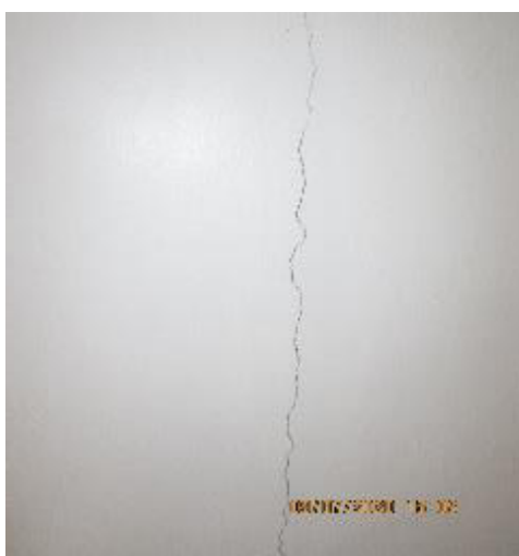
Photo 4.4(b): Showing Vertical cracks thru walls thickness at Santilya Health Centre in Mbeya DC. Photo was taken by the Auditor on 7 th July, 2020
