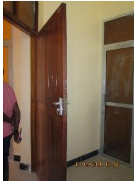
Photo 3.5 (b): Showing improperly fixed door which overlaps at Nzovwe. Photo was taken by Auditors on 7 th July, 2020 at Mbeya CC
