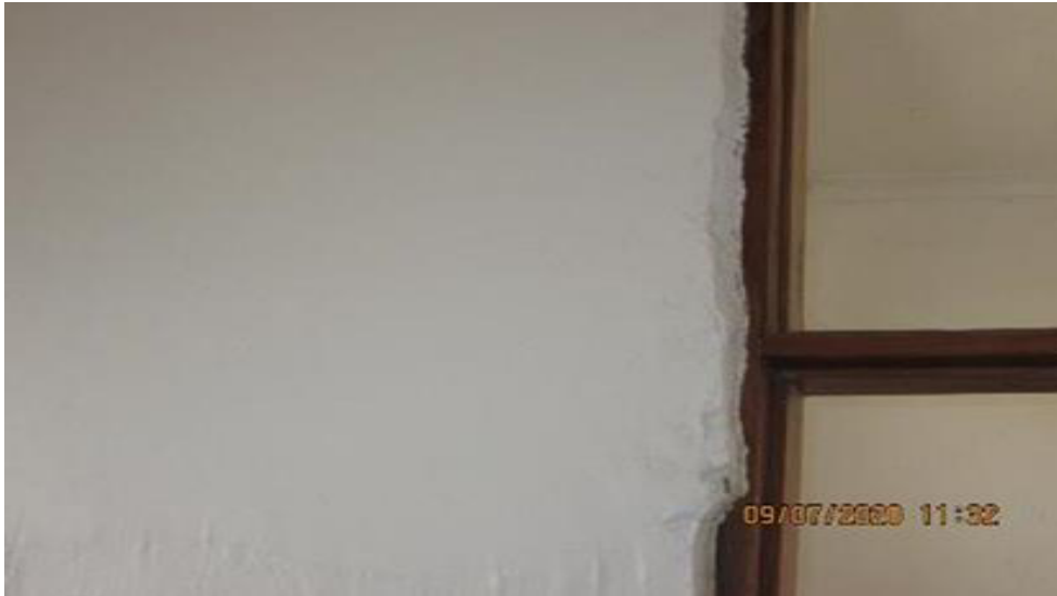
Photo 4.3: Shows Poor Workmanship of door opening at Mbeya District Hospital in Mbeya District Council (Photo taken by the Auditor on 09 th July, 2020)
