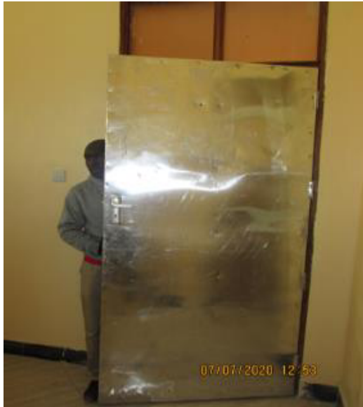
Photo 3.5(a): Showing improperly used x-ray shield in radiology room at lyunga. Photo was taken by Auditors on 7 th July, 2020 at Mbeya CC
