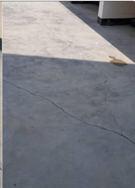
Photo 3.13: Floor cracking at dhobi area of Hostel building at Bulunde SS in Nzega TC.
