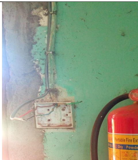
Photo 3.20: Electrical conductor or wire is bare at a switch near fire extinguisher in one of the buildings at Mpwapwa TTC.
