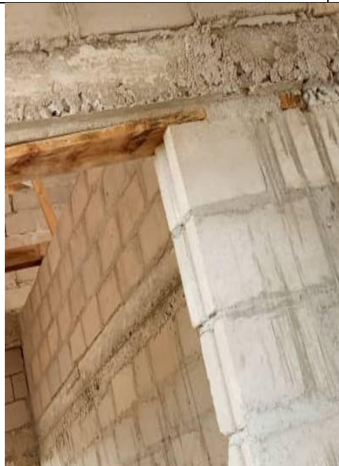
Photo 3.8: Ring beam having honey combs at multipurpose hall building at Kitangili SS In Nzega TC.
