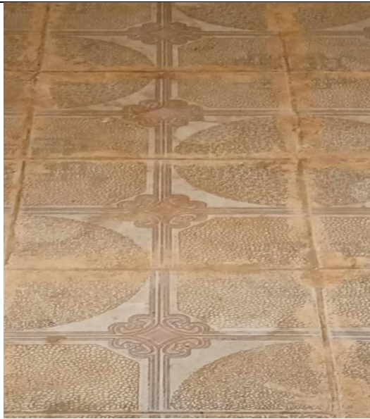
Photo 3.32: Floor tiles at the toilet area of the hostel at Nachingwea Girls SS not well grouted.
