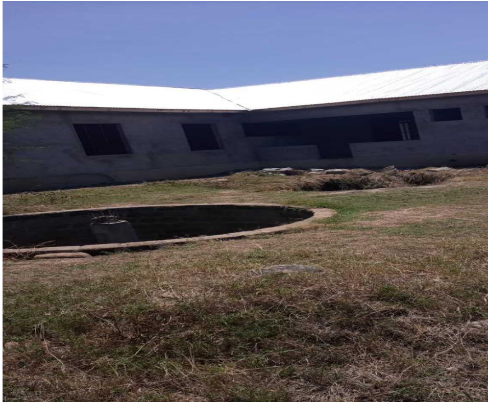
Photo 3.4: Uncovered Soak pit at Simiyu SS at Bariadi TC
