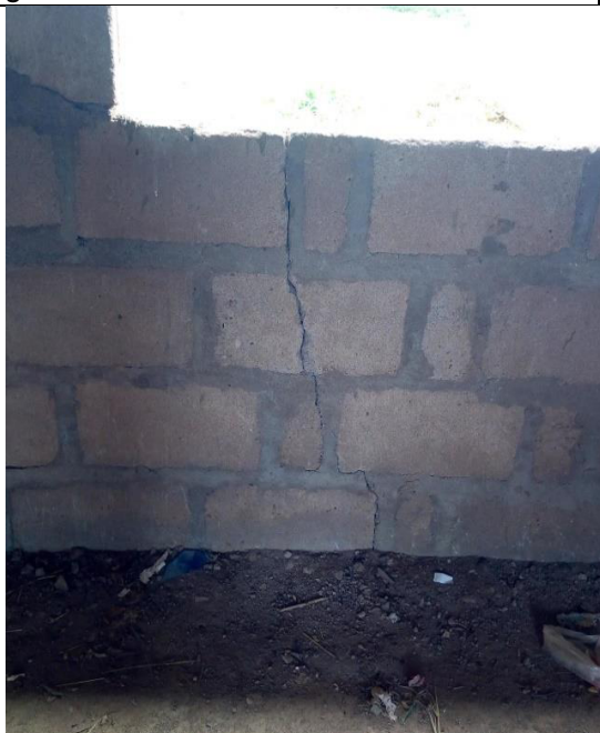
Photo 3.34: Wall crack at hostel building at Mazae Hostel Building
