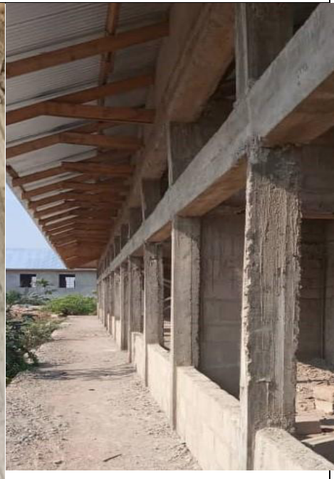
Photo 3.9: Columns of multipurpose hall at Kitangili SS un-straightened as required in Nzega TC.
