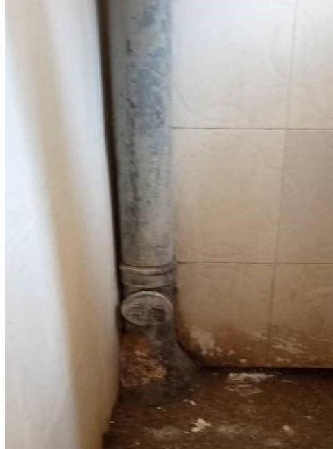
Photo 3.6: Waste pipe having leakage at one of the toilets at Klerruu TC
