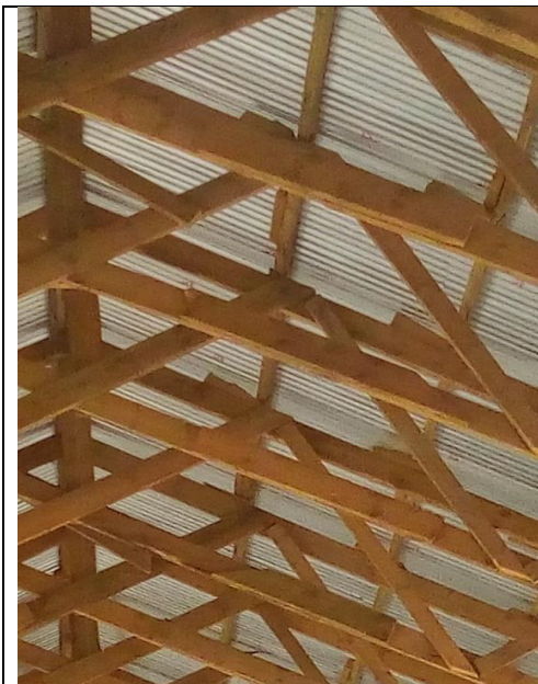
Photo 3.16: Roof trusses members jointed with unsatisfactory number of nails one or two
