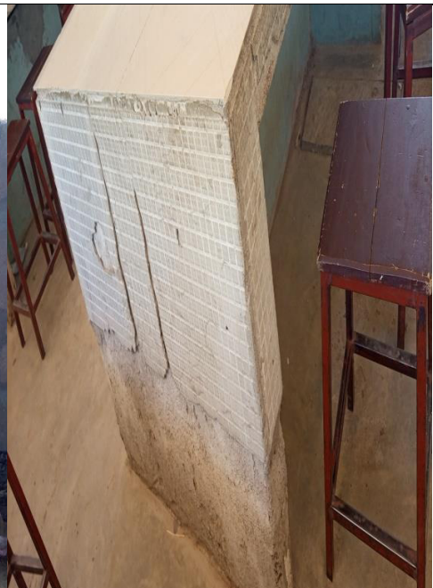
Photo 3.35: Wall tiles of Laboratory tables peeled off
