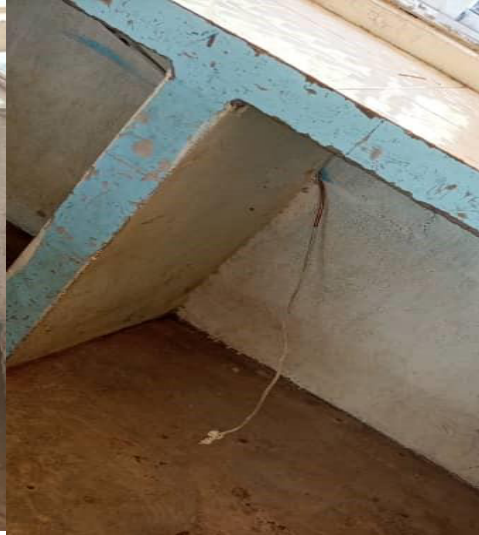
Photo 3.11: Gas system pipes hanging at one of the Laboratory rooms at Simiyu SS in Bariadi TC.
