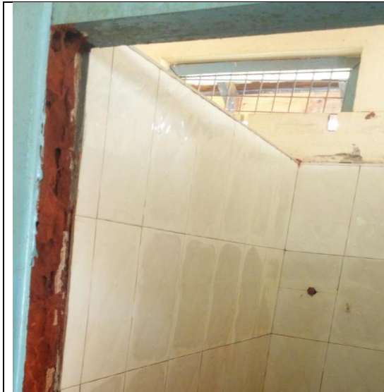
Photo 3.14: Door frame termite attack at Mpwapwa TTC.
