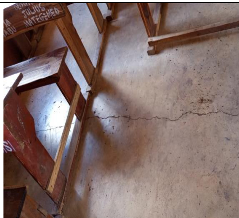
Photo 3.27: Floor cracking in one of the classrooms at Sima B SS in Bariadi TC
