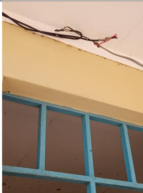
Photo 3.29: improper wire connection at Kidinda PS in Bariadi TC.
