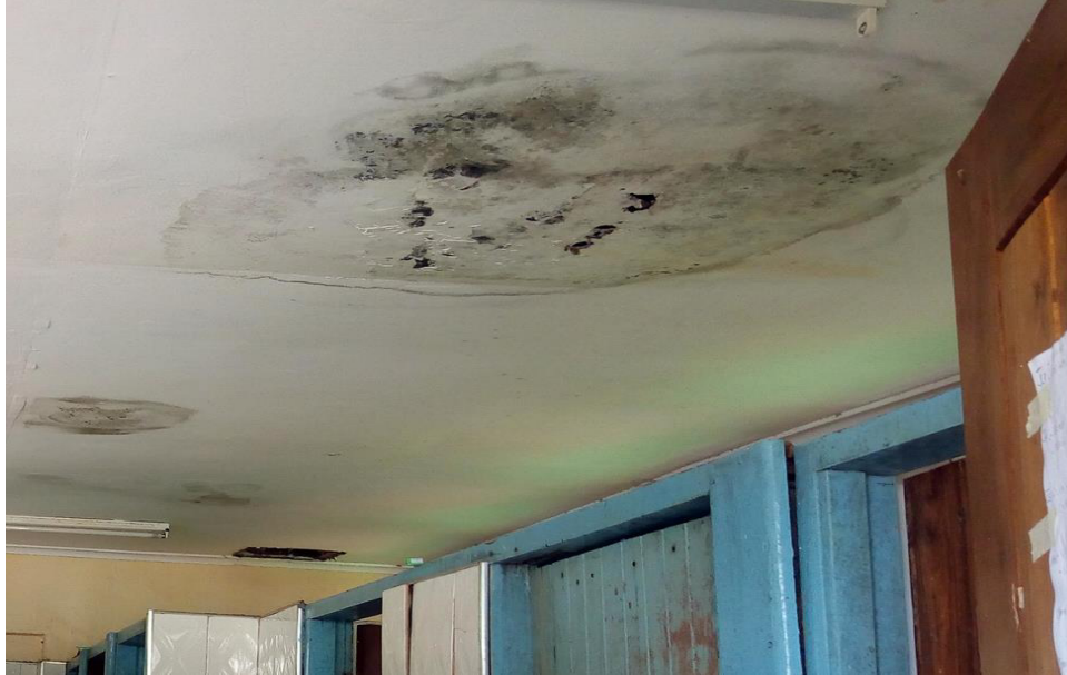
Photo 3.1: Roof leakage in one of the Dormitory ablution at Mpwapa Dormitories (Taken on 14 th January, 2021).
