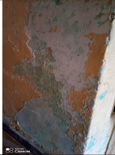
Photo 3.19: Peeling off of internal painting in one of the hostel building at Klerruu TTC.
