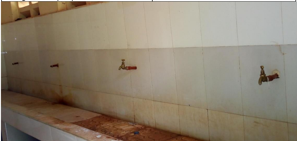
Photo 3.24: Unsustainability of water infrastructure: 2 out of 4 numbers of water corks had been removed at Mpwapwa TTC in Mpwapwa DC.
