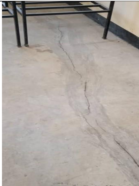
Photo 3.12: Floor cracking in one of the hostel building at Mwanzoli SS in Nzega TC.
