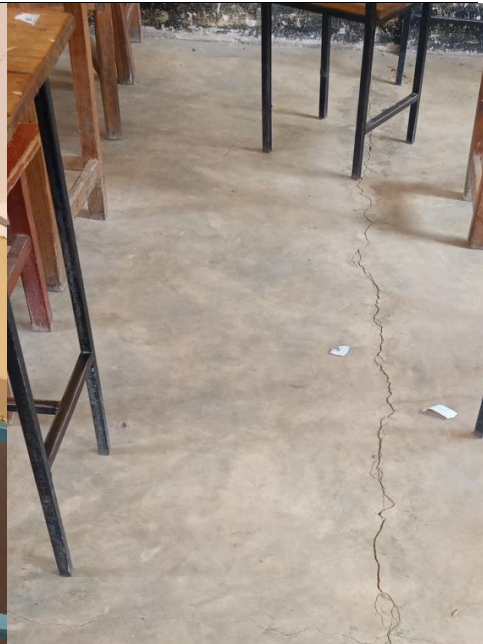
Photo 3.30: Floor crack in one of the classrooms at Tagamenda SS in Iringa MC.
