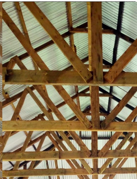
Photo 3.17: Roof trusses members jointed with unsatisfactory number of nails, one or two
