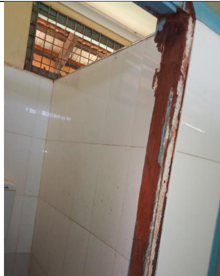
Photo 3.15: Door frame termite attack at Mpwapwa TTC.
