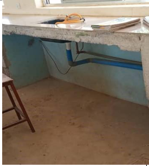
Photo 3.10: Wall tiles at Laboratory room removed off at Simiyu SS in Bariadi TC.
