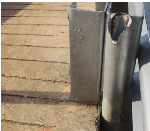
Photo 3.11c: Remaining piece post of stolen bridge chevron sign along Tanga-Horohoro road Ndoyo Bridge. Source: Auditors'
