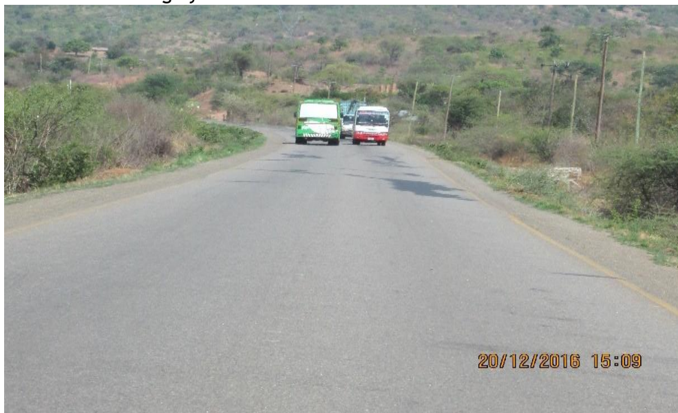
Photo 3.5 Worn out road markings along TANZAM Highway (Igawa-Mbeya) road captured by auditors on 20.12.2016
