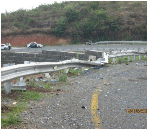
Photo 3.11a: Damaged guard rail along Mbeya-Lwanjilo-Chunya road. Source: Auditors'
