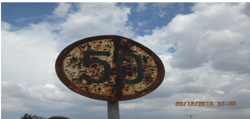
Photo 3.18: Corroded road sign captured by auditors at Chimala village as captured by auditors on 20/12/2016
