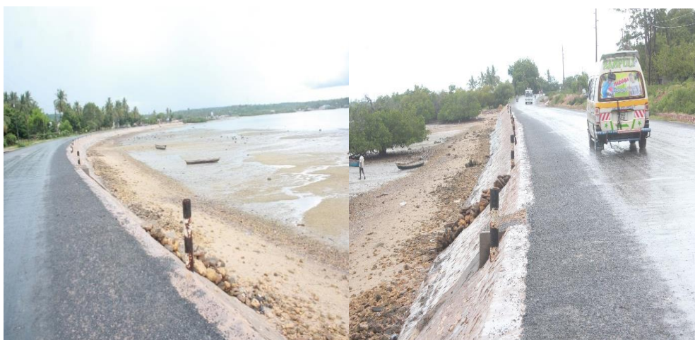
Photo 3.10 Missing guard rails along Kilwa road (Lindi-Mtwara) at Mikindani area in Mtwara. Photo taken by auditors on 17-Feb-2017
