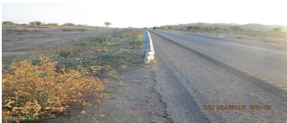
Photo 3.8 Protruding start of guardrail fishtail along Iringa - Dodoma road. Captured by Auditors on 16/12/2016
