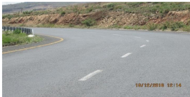
Photo 3.13c: Roads marking allowed overtaking in a sharp curve along Mbeya-Lwanjilo-Chunya road.
