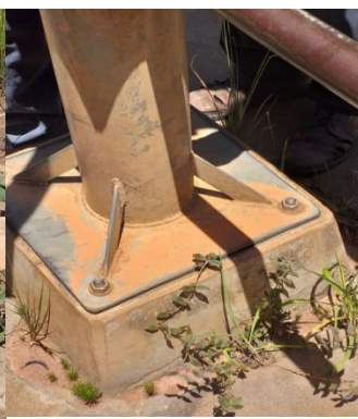
Photo 3.2b: Failed pump foundation as taken at Urambo on 15th February, 2019
