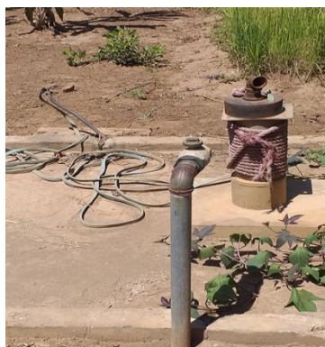
Photo 3.2a: Borehole with a failed pump due to electrical fault as taken at Relini area-Urambo on 15 th February, 2019
