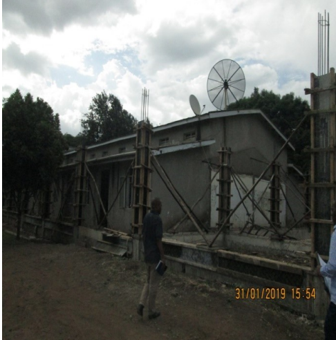
Photo 1.5: Building Permit # 514/2018, SDA Church in Arusha Region in Arusha Municipal Council under construction without structural design and drawings
