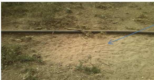
Photo 6.2: Pipe laid on the ground instead of being one meter below the ground
