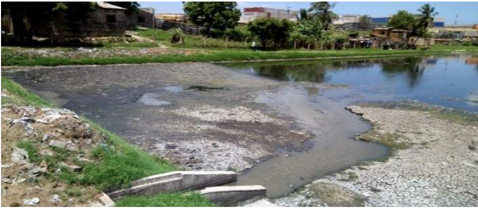
Photo 4.4(b): Showing a mixture of sludge and solid waste in anaerobic pond at Kurasini - Dar es Salaam (photograph was taken on 02 nd November, 2017)
