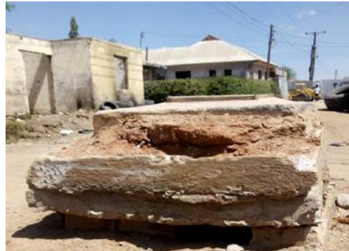
Photo 5.1: Blockage of pipes and destruction of sewer man hole at Kinyonga Street in Dodoma. Picture was taken on 06 th October 2017
