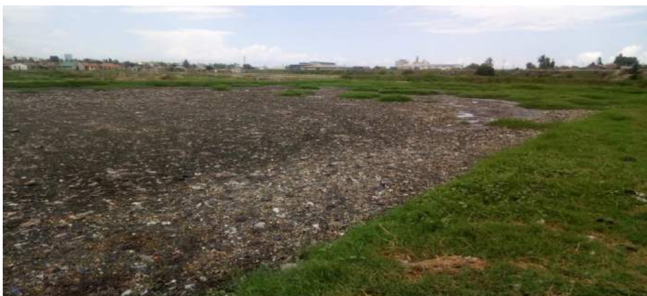
Photo 4.4(a): Showing an outer look of in-use Vingunguti anaerobic pond with a resembling of a solid waste dumping site(Photo was taken on 31 st October, 2017 at Vingunguti WSP).
