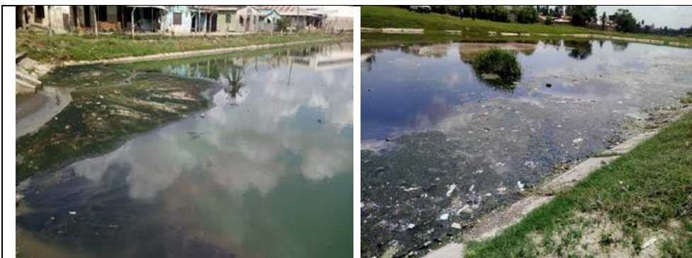
Photo 4.3(c): Buguruni Anaerobic Pond accumulated sludge (Photograph was taken on 1/11/2017 in Tanga)
