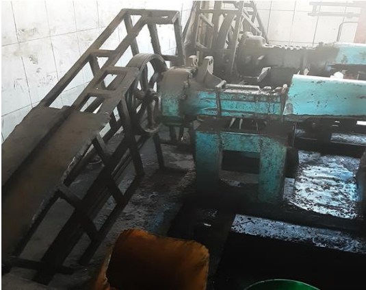
Photo 3.2(a): Inadequately furnished locally made Sunflower Oil pressing Machine, as taken by Auditors at Mbeya on 3 rd October,2022.
