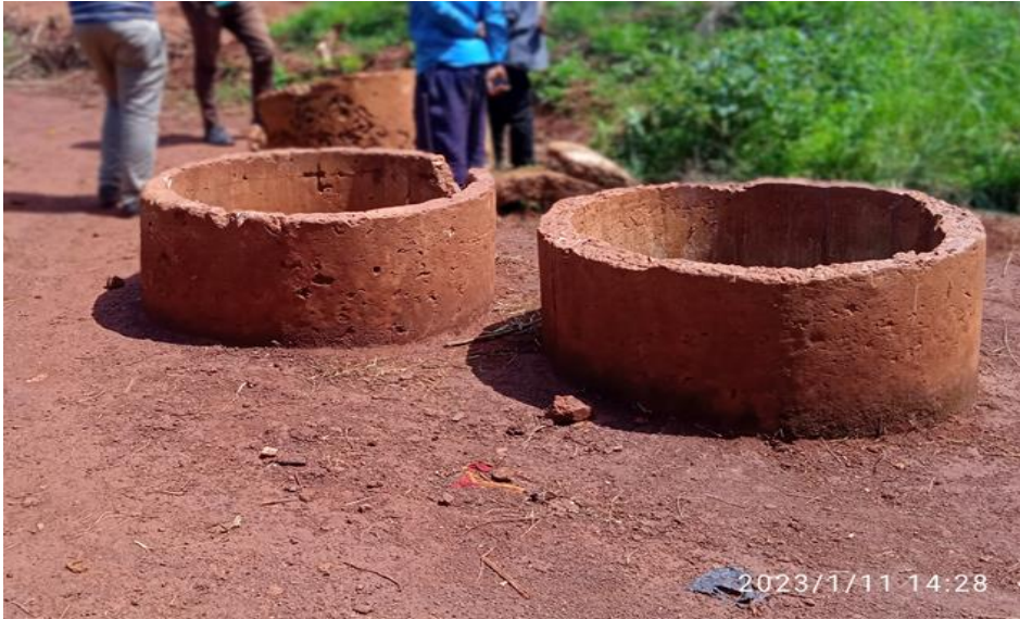
Photo 3.3: A Sample of abandoned boreholes at Uvinza PAA, Whereby the observed ring could not be inserted and joined by TASAF. The Photo was taken by the Auditors on 11 th January, 2023 at 2:28 P.M
