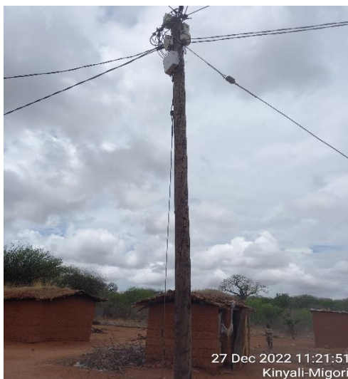
Photo 3.3: Wooden poles which did not have warning plates and the barbed wires.
