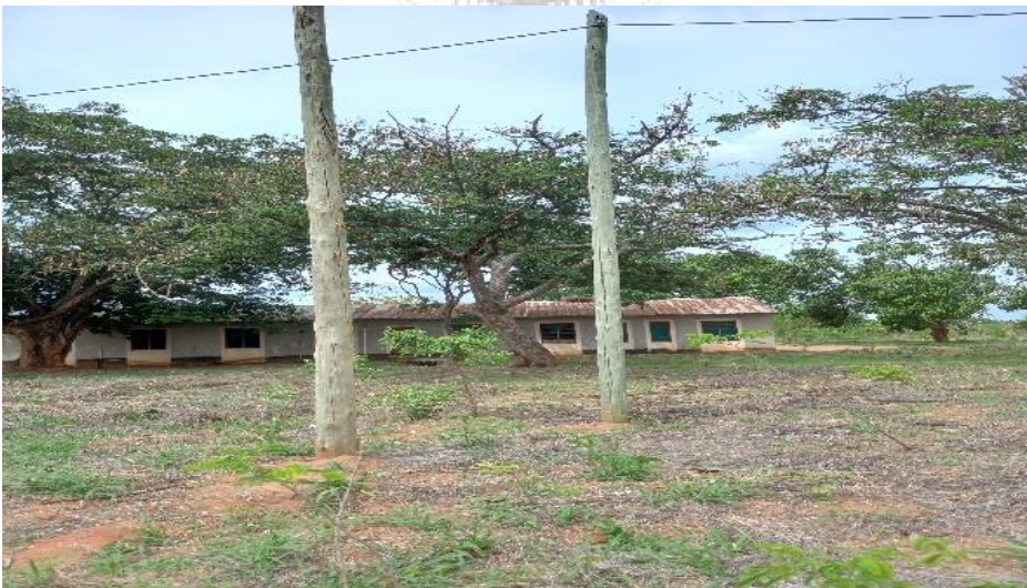
Photo 5.4: Unlabeled electric poles in all visited sites at Matekwe in Nachingwea DC. The Photo was taken by the Auditors, December, 2022
