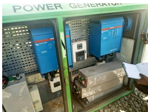
Photo 5.5 (a): Non-functioning batteries at Mavota Village - Biharamulo District, the Photos were taken by the Auditors on 29 th December, 2022
