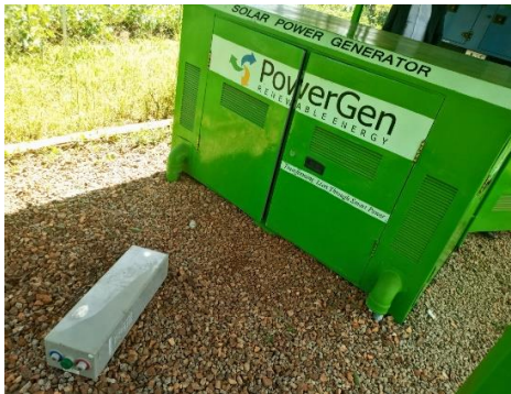
Photo 5.5 (c): showing non-functioning battery disconnected from other batteries placed on surface
