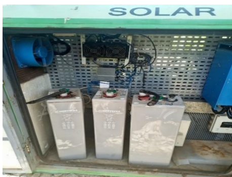
Photo 5.5 (a): Non-functioning batteries at Mavota Village - Biharamulo District, the Photos were taken by the Auditors on 29 th December, 2022
