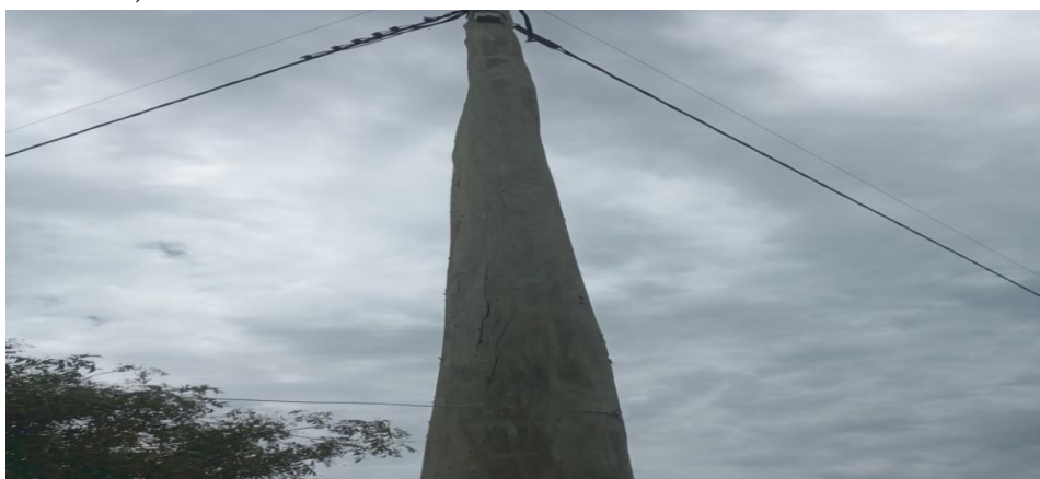
Photo 5.4: One of the poor quality electric pole (with cracks) installed by PowerGen in Iglansoni Village (Ikungi District in Singida). The Photo was taken by the Auditors on 22 nd December, 2022
