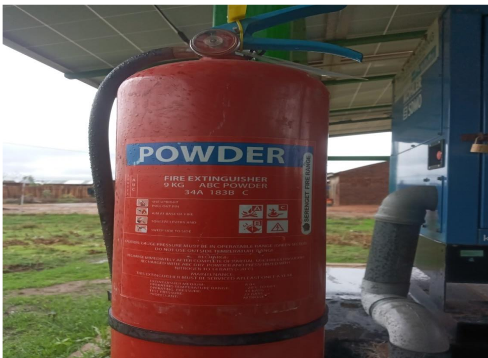
Photo 5.6: Fire extinguishers which had no maintenance label and was abandoned at site without replacement at Iglansoni Village in Ikungi District (Singida). The photo was taken by Auditors on 19 th December, 2022
