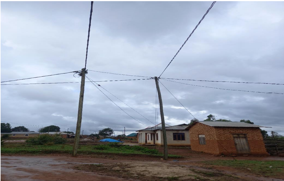
Photo 5.1: To the Left: TANESCO's Electric Pole: To the Right; Project Developer's Pole both supplying electricity to a single house hold at Kifumbe Village in Makambako District Council. Photo taken by Auditors in 28 th December, 2022
