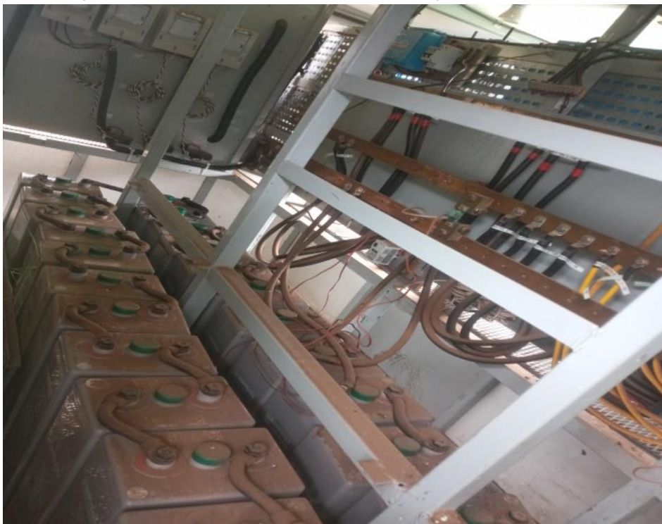
Photo 5.5.4: Depleted batteries due to non-maintenance and abandonment at Iglansoni Village Power plant. Photo was taken by the Auditors on 22 nd December, 2022.
