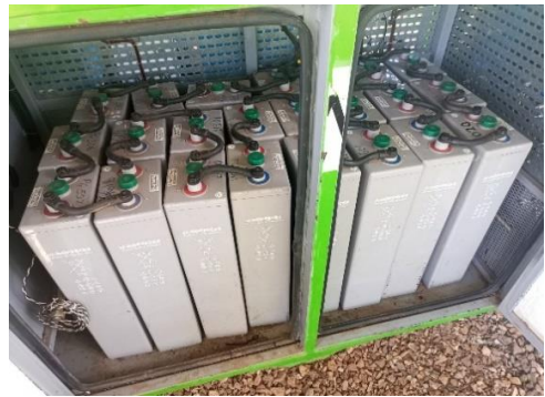
Photo 5.5 (d): showing 23 batteries connected however they are not functioning
