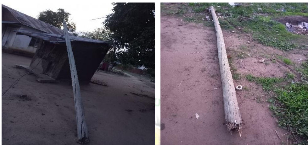
Photo 5.6: Broken electric pole at Nanjilinji Village as it was observed by the Audit Team during the Site Visit on 20 th December, 2022
