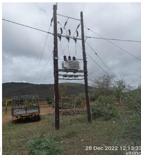
Photo 3.3: Wooden poles which did not have warning plates and the barbed wires.
