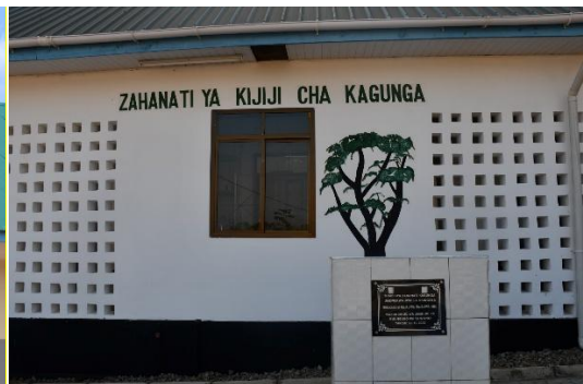
Photo 3.2: Constructed Health Centre at Kagunga Village, Photo taken by Auditors during a Site Visit at Kagunga Village on 19 September 2024
