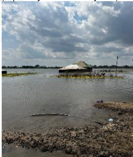
Photos 3.3(d): Residential areas invaded with water in the lower part of Muhoro Ward in the Rufiji District along the Rufiji River. (Caption by Auditors as of July 2024)
