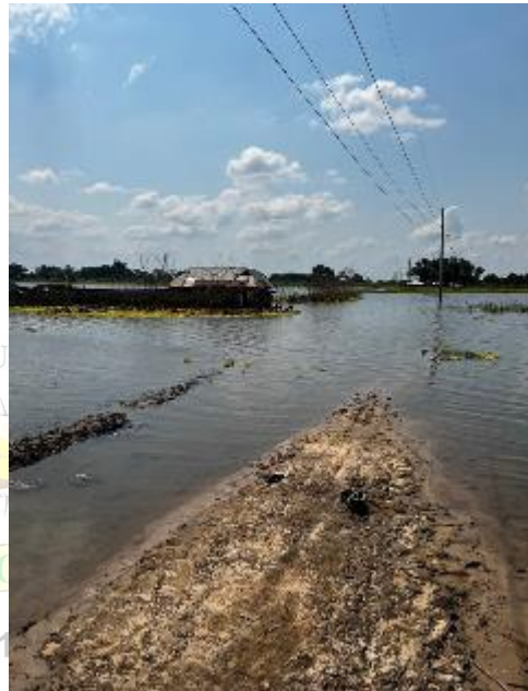
Photo 3.2(b): Residential buildings, roads, and electrical infrastructures were invaded by flood waters caused by water overflow over the river banks along the flood-prone areas of Muhoro Ward in the Rufiji District along the Rufiji River.
