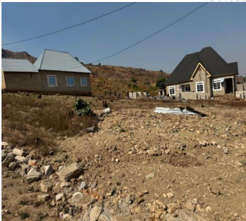
Photo 3.5 (a): showing uncompensated residential houses close to mudslides at Itezi-Mbeya (Caption by Auditors in September 2024)
