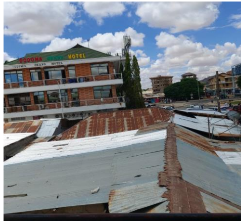
Photo 3.2: Non-compliance to Master Plan - Dodoma CC 10 th Street. (Auditors' Caption on 22 nd September, 2023)
