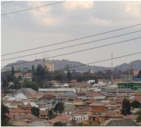
Photo 3.1: Non-compliance with Master and detailed plans at CBD in - Iringa MC (Market, Kihasa, Uhindini, Old bus terminal and Ilala Streets) (Photo taken by Auditors on 29 th September, 2023)
