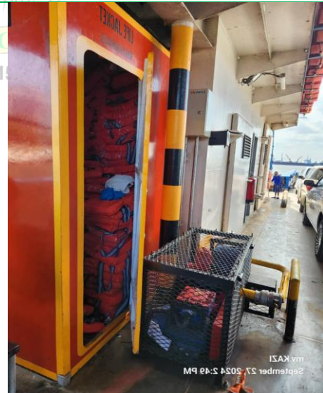
Photo 3.7(d) , Fuel system obscured life jacket cage on MV Kazi
