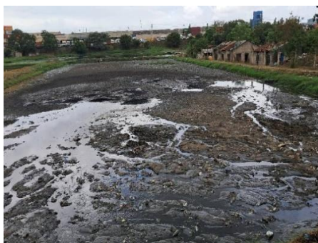
Photo 3.1: Waste Stabilisation Pond at Kurasini in Dar es Salaam requiring desludging
