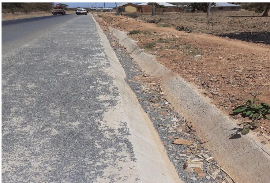
Photo 1: Chipping strip-off as one of the defects along Don-Bosco Mawelewele Road in Iringa MC.
