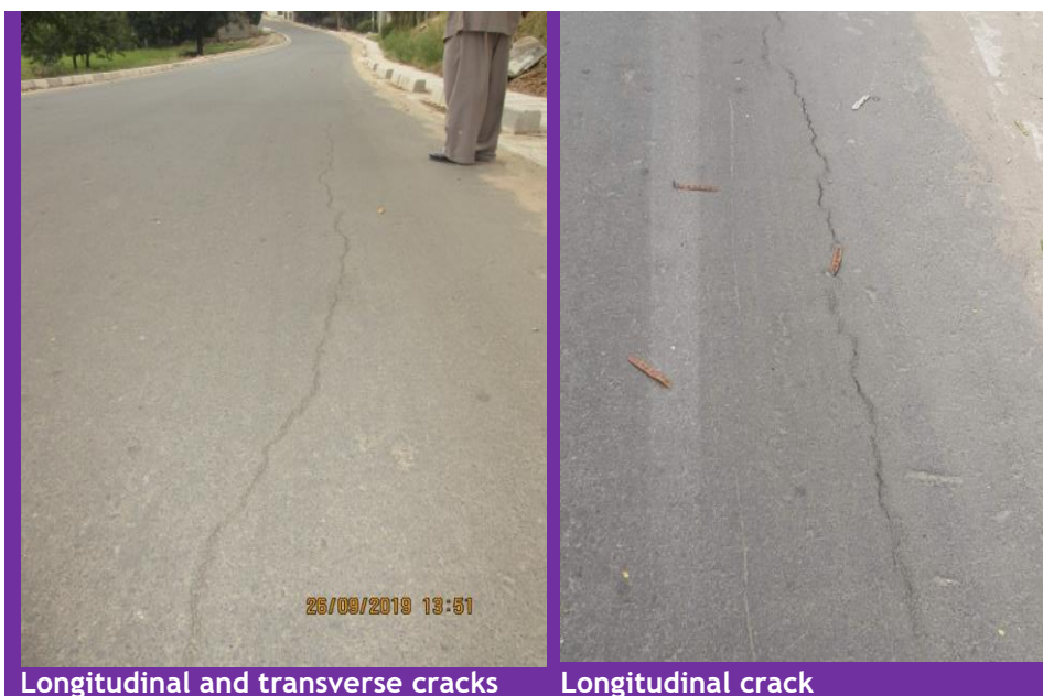
Photo 3: Longitudinal and transverse cracks observed along Changanyikeni-Shule Road (Photo taken by auditors on 26 th Sept 2019)
