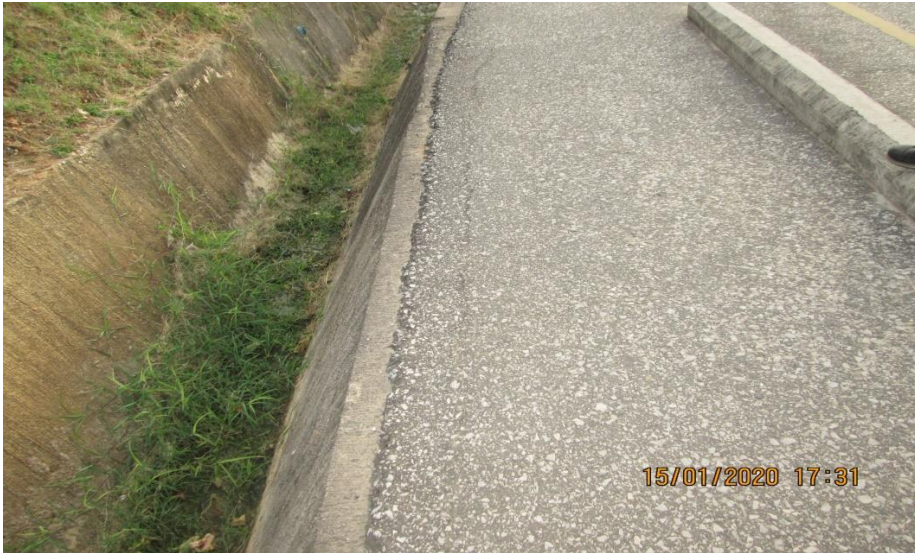
Photo 2: Coral limestone aggregates used for wearing course mined from the wrong sources as per original design. (Photo taken by auditors on 15th January 2020)
