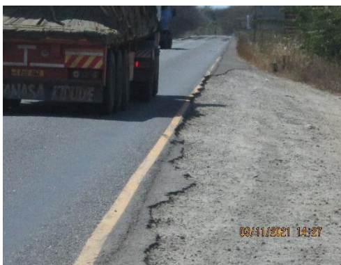
Photo 3.1: Loss of shoulder width along Morogoro Dodoma Road (caption of 03 rd November, 2021)
