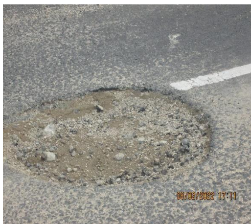
Photo 3.3: Pothole observed along the centerline and carriageway of Gehandu - Babati Road (Caption of 08 th February 2022)
