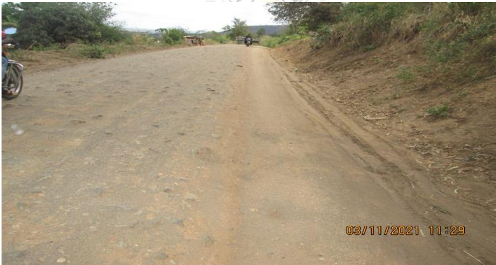
Photo 3.3: Shows badly affected Bigwa - Kisaki Road with defects (Stoniness) and traffic-ability on shoulder (Caption by Auditor on 03 rd November 2021)
