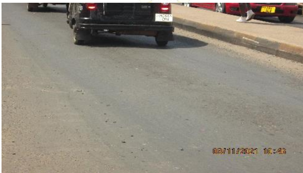
Photo 4.1: Shows Msamvu-Morogoro roundabout -Bigwa Junction with defects of strip-off chippings, bleeding and rutting (Caption by Auditors 3 rd Nov 2021 at 10hr48).
