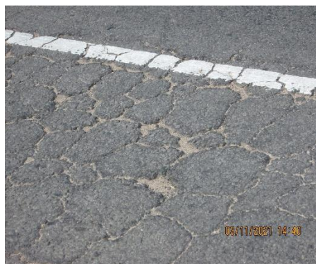
Photo 3.2: Alligator cracks along Morogoro Dodoma Roads (caption of 03 rd November, 2021)
