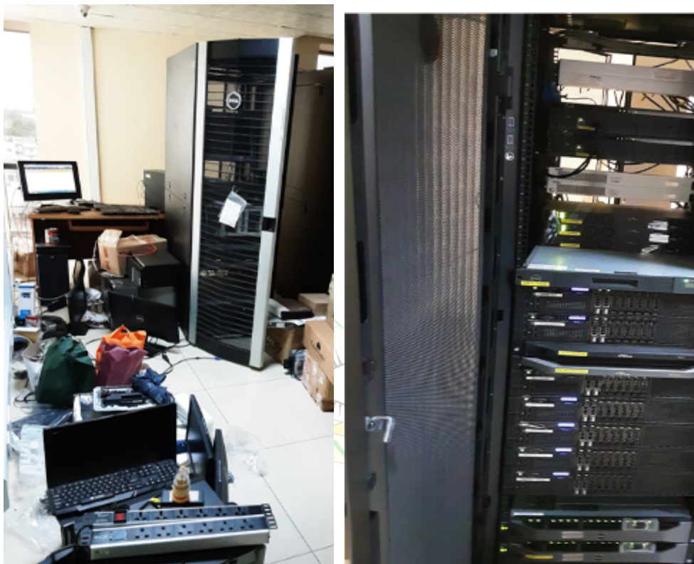
Photos 3.1 (a) and (b): Servers in a server room (Primary Site) stacked together with other irrelevant luggage contrary to server room requirements. Photo taken by Auditors on 29 th October, 2021
