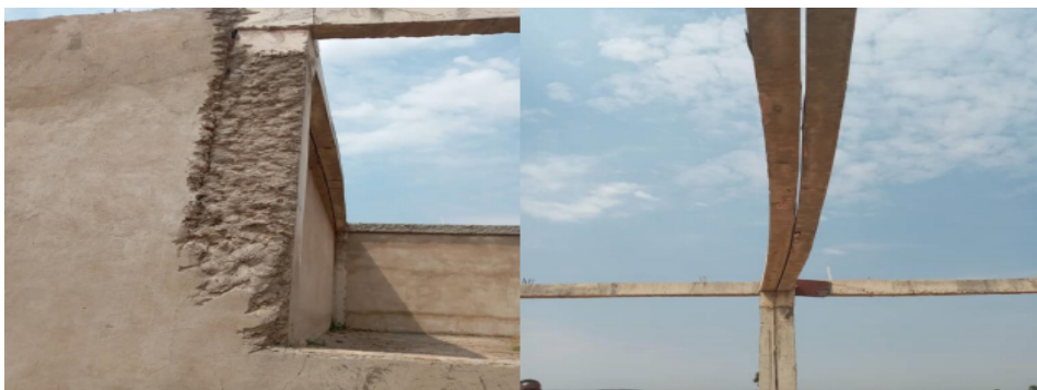
Photo 3.1: Cracks in the Joints between the walls and the pillars in the floor, Curved beam, poor grip of plaster, concrete cracks for columns and beams
