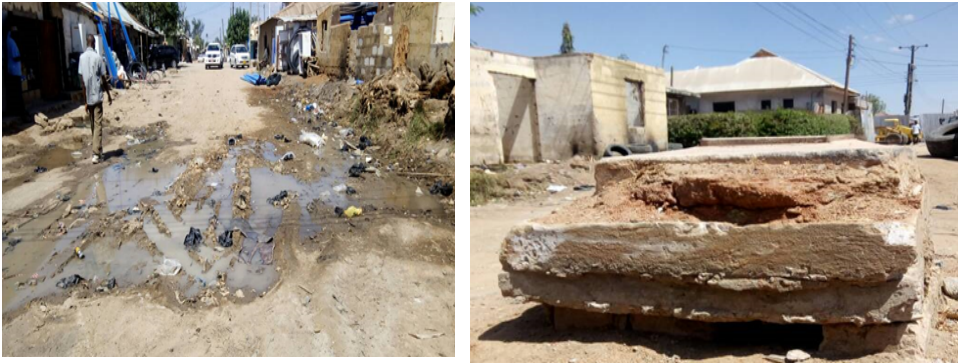
Photo 5.1: Blockage of pipes and destruction of sewer man hole at Kinyonga Street in Dodoma. Picture was taken on 06 th October 2017
