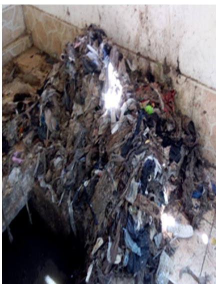
Photo 4.2 (a): Showing Solid material removed from sewer network: (Photograph was taken on 31/10/2017 in Tanga)
