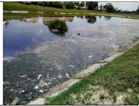
Photo 4.3 (d): Mabibo Anaerobic Pond accumulated sludge and bushes (Photograph was taken on 1/11/2017 in Tanga)
