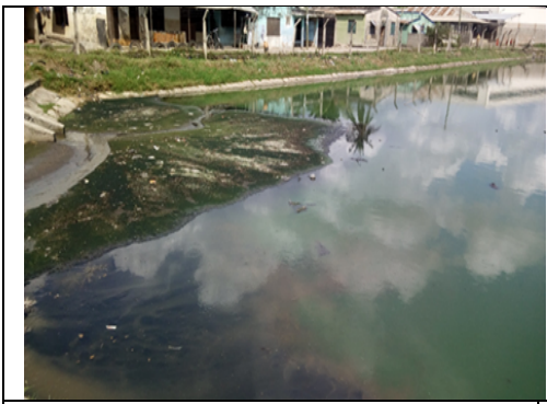
Photo 4.3(c): Buguruni Anaerobic Pond accumulated sludge (Photograph was taken on 1/11/2017 in Tanga)
