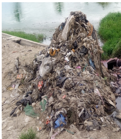
Photo 4.2 (b) Showing Solid material removed from sewer Network: (Photograph was taken on 31/10/2017 at Vingunguti Ponds in Dar es Salaam)
